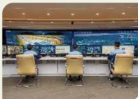
■ Huangge Water Plant’s “Smart Brain” – Central Control Room
