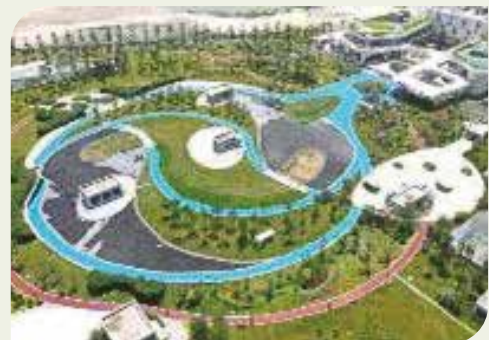
■ The Park-Style Design of Water Holdings’s Shanwei Eastern Water Purification Plant
