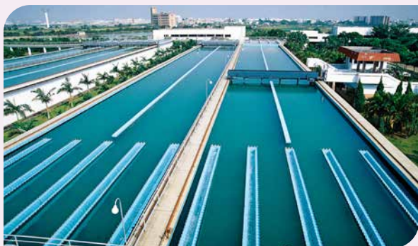
■ Shantou Water Plant
